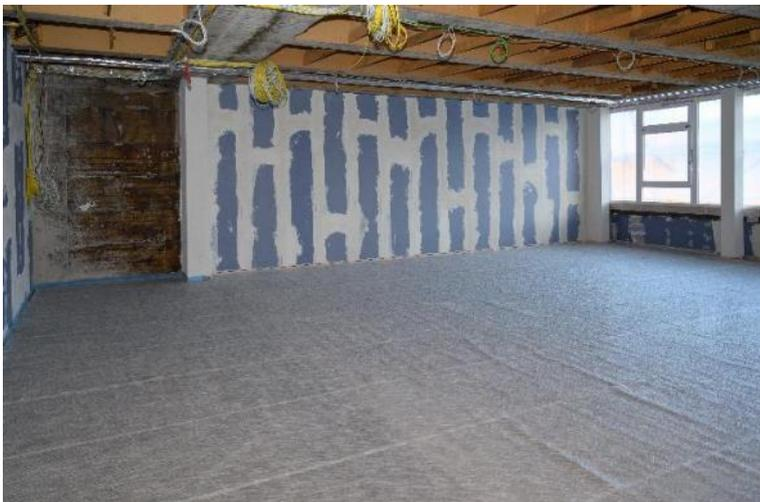
Complete refurbishment of the Löffingen secondary school: With the recommendation from PCI and the appropriate PCI products, the floor was laid on a critical substrate without dismantling the dilapidated screed.
