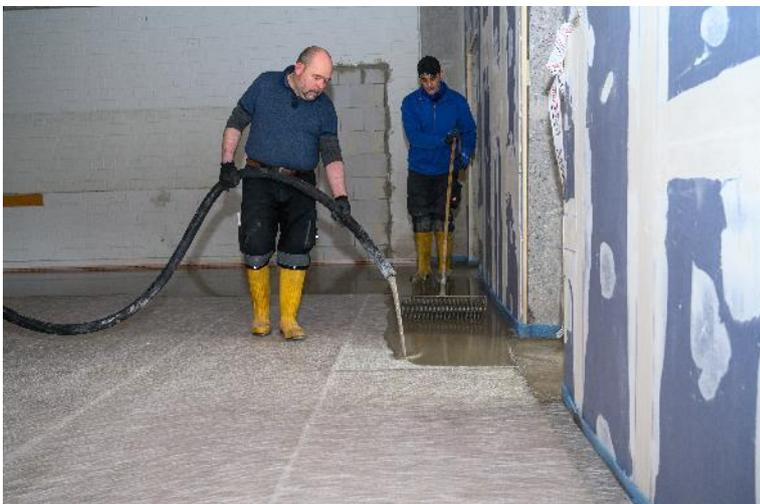
After priming with PCI Gisogrund 404, the craftsmen laid out the glass fiber reinforcement PCI Armiermatte GFM and spread the special leveler PCI Periplan Extra on top.
