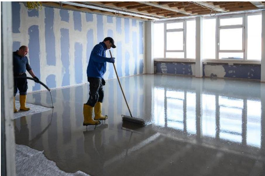
*Easy processing, fast construction progress: PCI Periplan Extra is self-leveling and can be walked on after around three hours. (Link to the high-resolution [Photo](#))*
