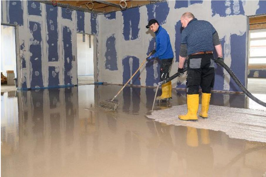
*Reliable floor structure: glass fiber reinforced bonded floor leveling with PCI Amiermatte GFM and PCI Periplan Extra (link to the high-resolution [Photo](#))*
