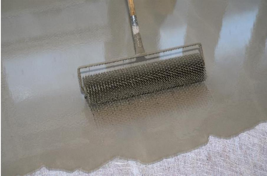
The low-dust and very low-emission floor leveler PCI Periplan Extra is suitable for layer thicknesses of 3 - 60 mm. (Link to the high-resolution [Photo](#))
