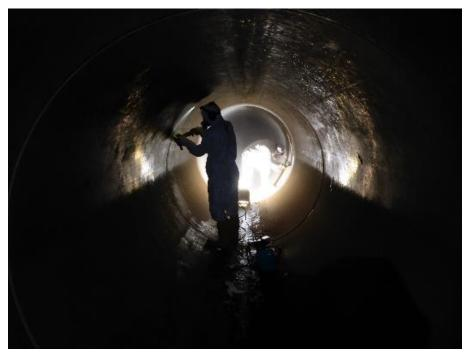
Leaky joints in a pipe route below Ebertstraße between Potsdamer Platz and the Brandenburg Gate: STRABAG AG refurbished 84 socket joints with PCI products. (Link to high resolution <u>Photo</u>)
