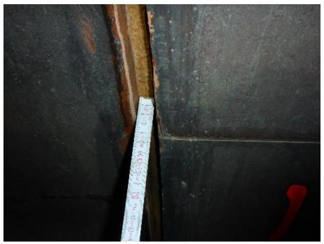
The joints were dismantled and cleaned, the joint depth was measured. (Link to high resolution <u>Photo</u>)
