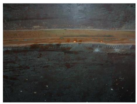
The joints were moistened on the back in many places. (Link to high-resolution <u>Photo</u>)
