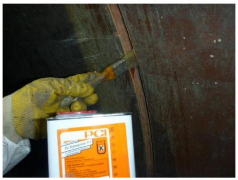
For a reliable 2-flank adhesion, the adhesive primer PCI Elastoprimer 110 was applied to the inner edges of the joint and the PE backing material DIN Polyband was pressed into place. PCI Escutan<sup>®</sup> TF was used as a polyurethane sealant to re-seal the 84 socket joints. (Link to high resolution <u>Photo</u>)
