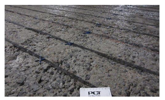
The anode strips are laid according to the architect's specifications on the concrete substrate prepared with ultra-high-pressure water jetting and mechanically fixed.
