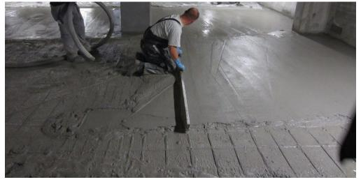
The fresh mortar is installed "fresh in fresh" into the mortar bonding agent while still fresh. This requires a great deal of attention from the processor. This is because the anode network or the cable tapes of the CCP system are embedded in the fresh mortar bed during this process. Later, current flows through the anode network, which is needed for corrosion protection of the reinforcing steel.
