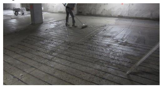
The anode tapes which were fixed in strips on the floor to be coated are clearly visible. A bonding agent made of the concrete repair mortar PCI Nanocret R4 SA's own material is applied to the matt damp substrate. Subsequently, the fresh mortar is installed "fresh in fresh" into the mortar bonding agent while still fresh.
