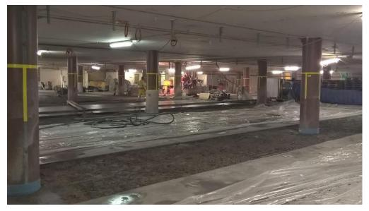
Mixing mortar, pumping, leveling and, according to the specifications of the architects, finishing the surface for the subsequent parking deck coating.
