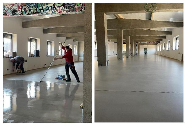
The sealing PCI Zemtec Top gives the directly usable concrete surface a silk matt, optically attractive surface. (Links to the high-resolution photos: <u>left</u>, <u>right</u>)
