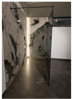
The large format tiles were laid with PCI FT Flex and PCI Flexmörtel S1 Flott. (<u>Link</u> to high-resolution photo)
