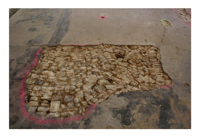
Historical paving was located under the existing screed, which was present in various qualities. This paving needed to be retained under all circumstances. After the necessary removal of damaged areas, the construction professionals were able to re-profile the substrate.
