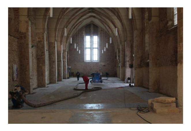
All bonding-inimical coatings and contamination were removed by the workers using steel ball shotblasting before re-profiling the defective areas with a stable repair mortar.
