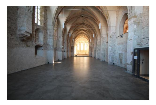
To complete the floor renovation, the dispersion-based sealing PCI Zemtec Top was applied as a glaze. This achieved a variegated surface appearance. In addition, the substrate in the Franciscan church is now anti-skid and wear-resistant - and ready for future events.
