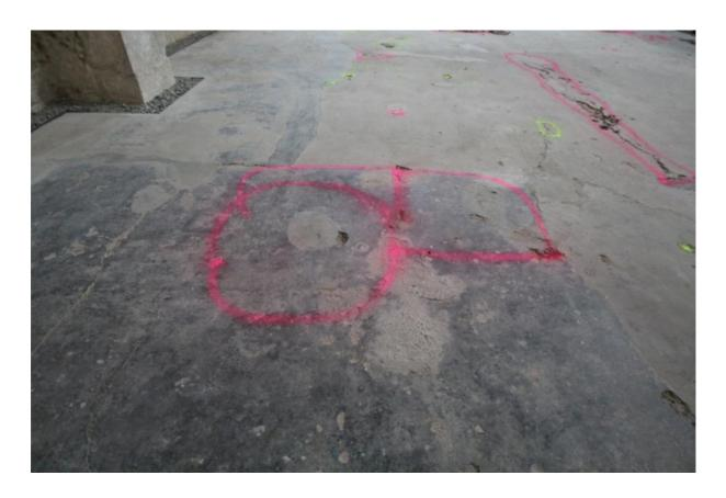
The preparatory work for the floor renovation in the Franciscan church included the marking of defects, extensive hollow layers and cracks in the substrate. This ensured that no damage was overlooked.
