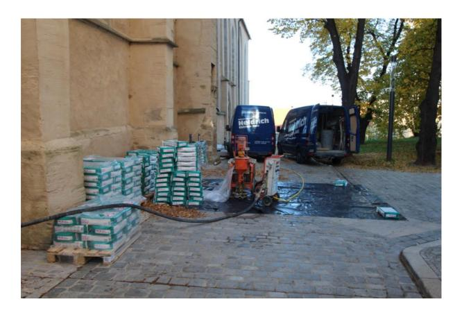
The team, under Andreas Heidrich, processed in total around eight tonnes of the cement-based floor leveller PCI Zemtec 1K. In order to achieve a high work output, the workers pumped the product into the interior of the church.
