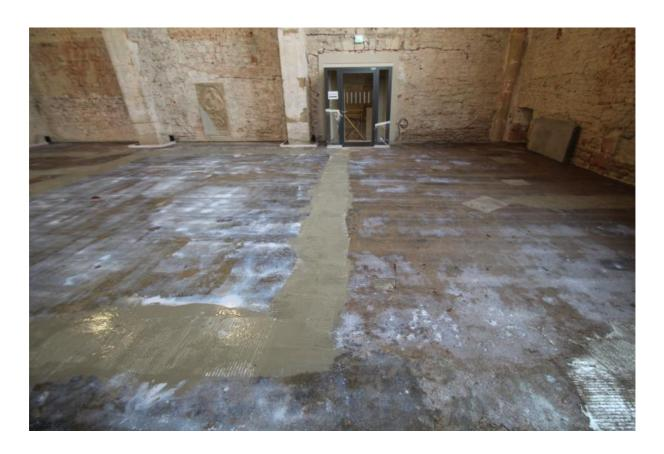
The special wash primer PCI Gisogrund 404 was applied to the re-profiled floor in two layers. The violet control colour of the synthetic resin dispersion enables precise application. This allowed the construction professionals to create a solid adhesive bond for the next layer.
