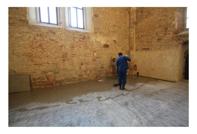
The construction professionals smoothed and removed the air from the floor levelling compound with the help of spiked rollers. As the product flows easily, it can be simply processed with little work outlay.
